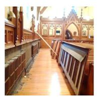
In mid-August, the pews were moved and the wood panelling removed to get at the asbestos behind the radiators. We found some old stencilling there as well.
